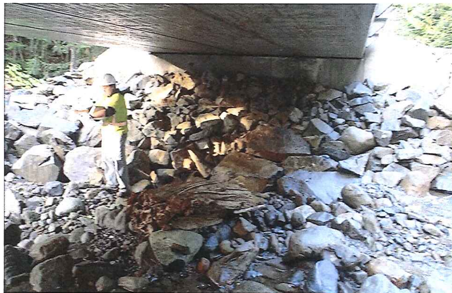
CK2466 Right Abutment
