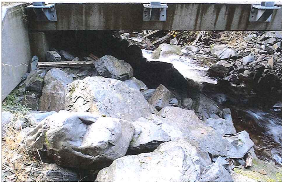
CK2466 Left Abutment Riprap
