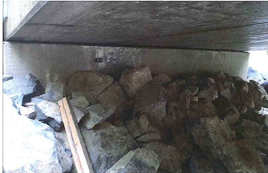
CK2466 Left Abutment
